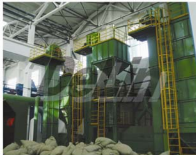
砂处理设备 Sand Preparation Equipment
